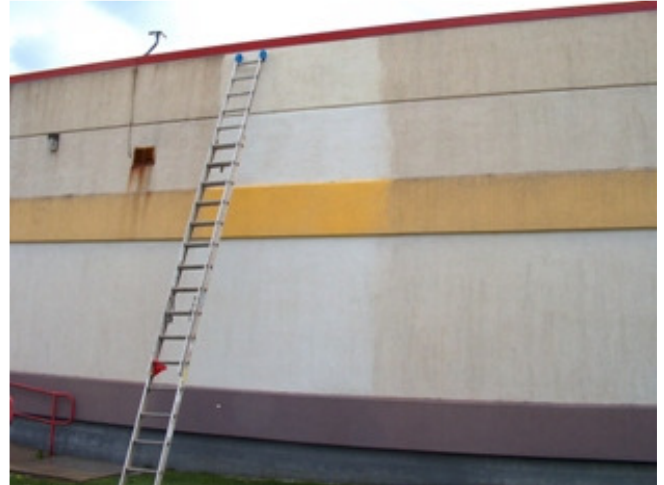
Before/After Using SB 2600 on EIFS Test Panel for Project
